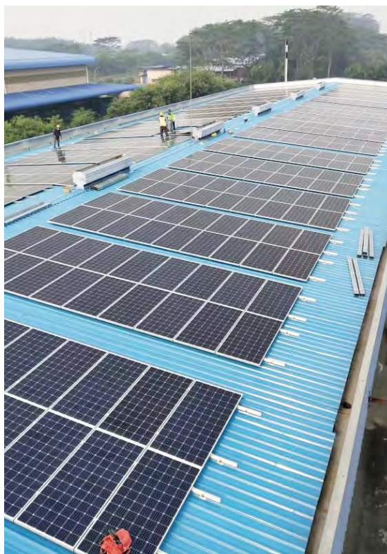
Trapezoid Metal Roof 200KW
