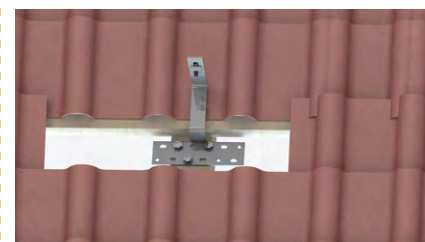
Drill a hole on the roof, then fasten the Hook to the hole by screw
