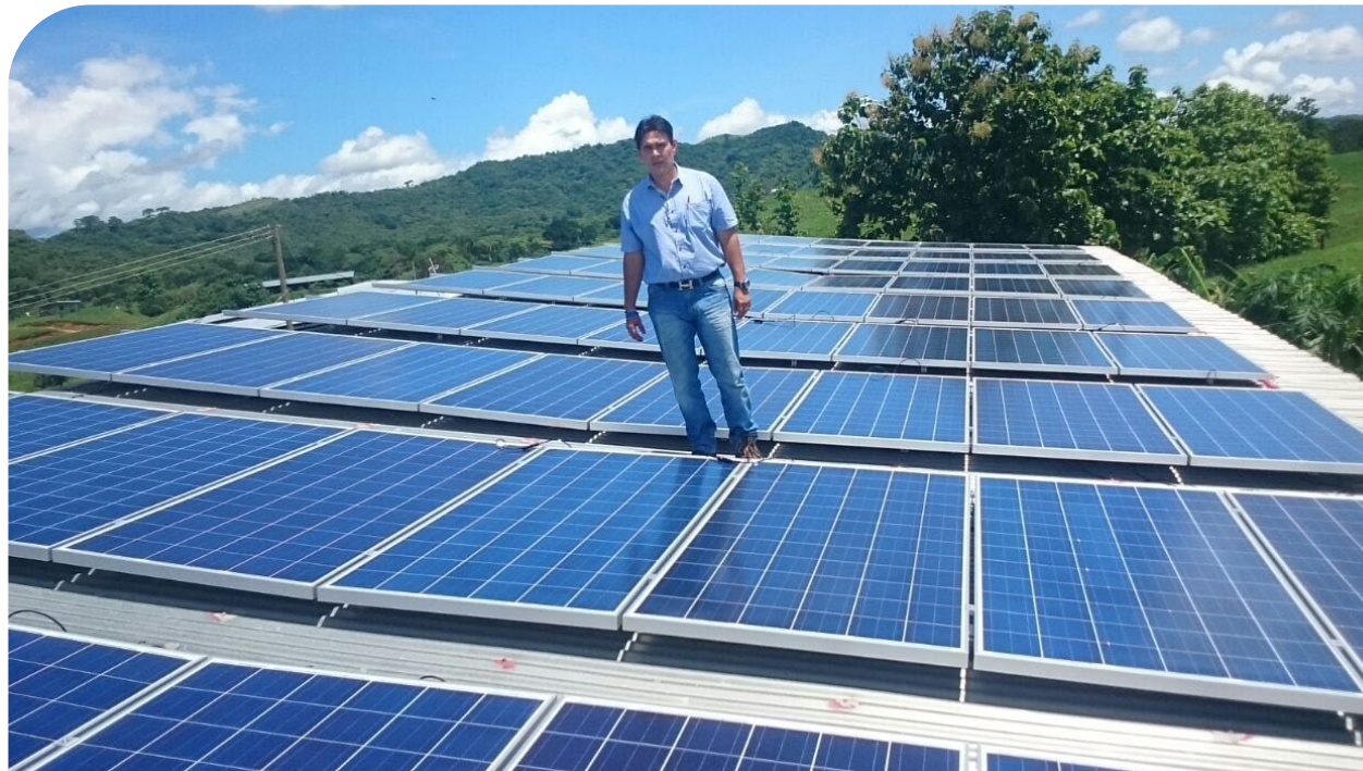
Panama 100KW Metal Roof
